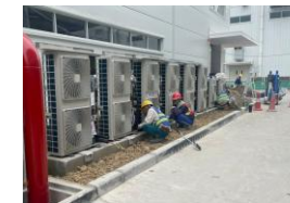
Outdoor unit installation work
